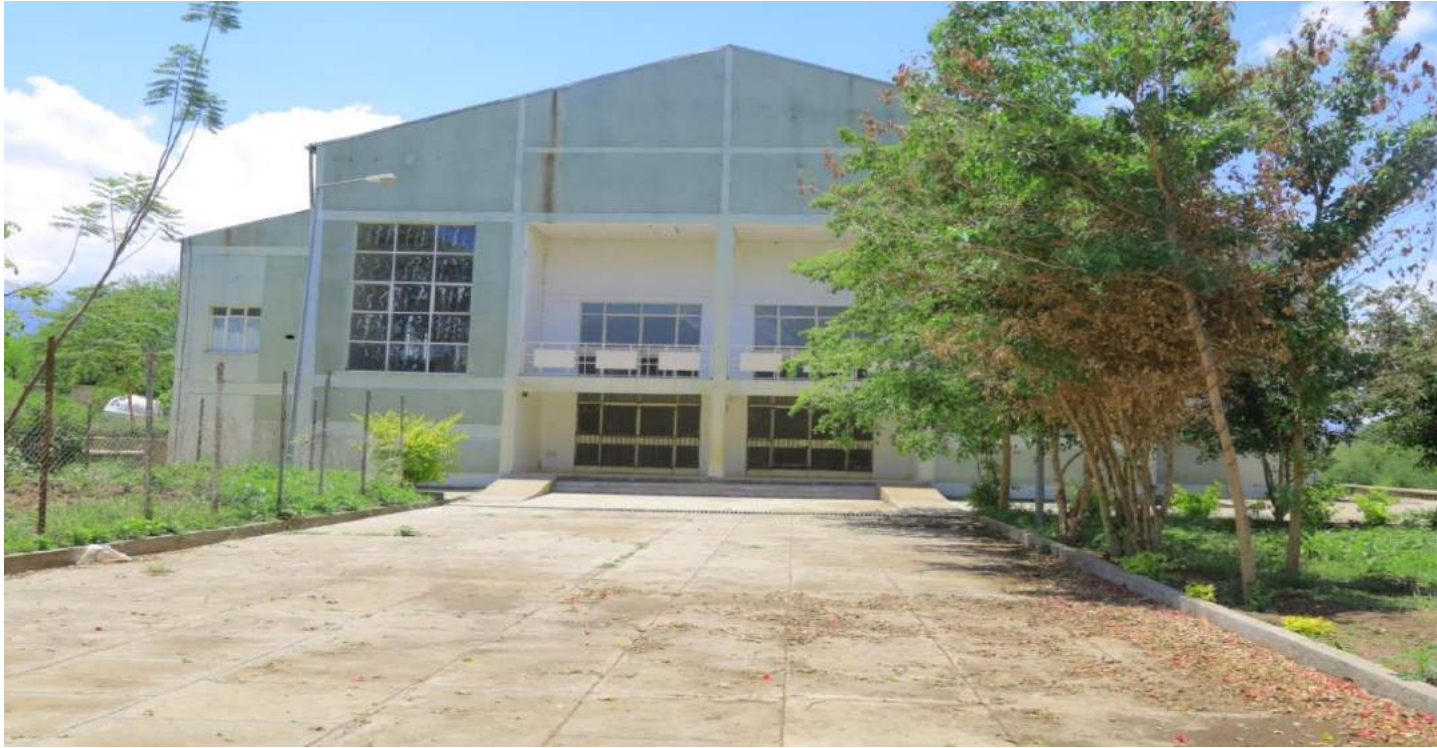
GYM N° 1, Main Campus
